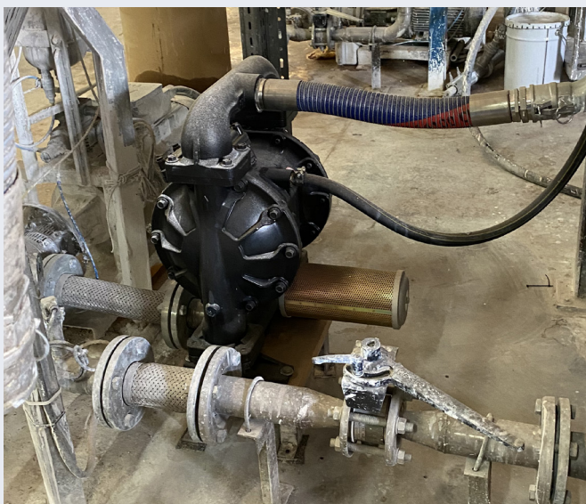
High suction lift reduces pump delivery.
